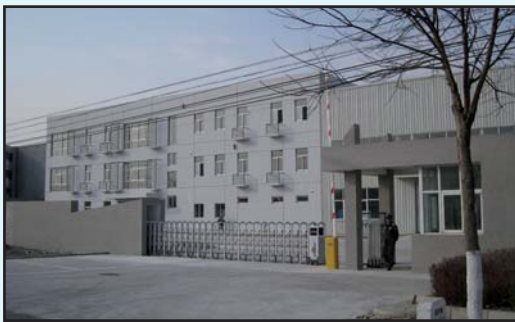
Left and below: The new JC-Tadano hydraulic components factory in Beijing
