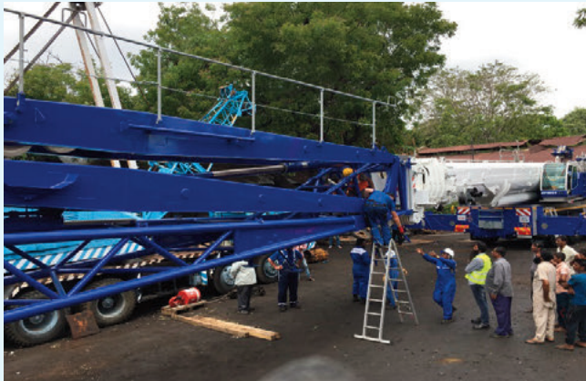
Tadano India commissioned Modern Cranes' ATF 400G-6
