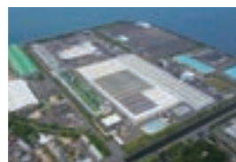
Solar panels installed at Shido Plant
