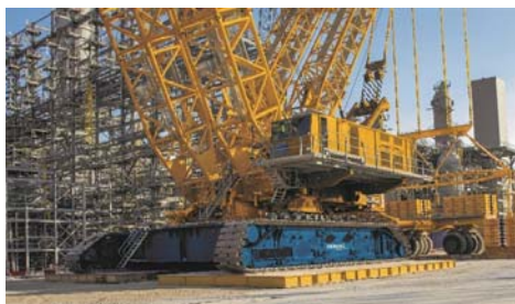
Demag Crawler Crane
