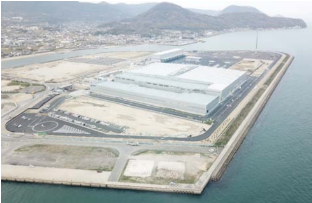
New plant viewed from the east (March 2019)
