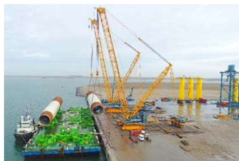
Crawler cranes loading offshore wind turbine components at a port
