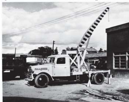
The OC-2 hydraulic truck crane
