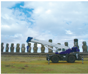
Moai Restoration Project
