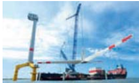
Assembling equipment in the harbor
