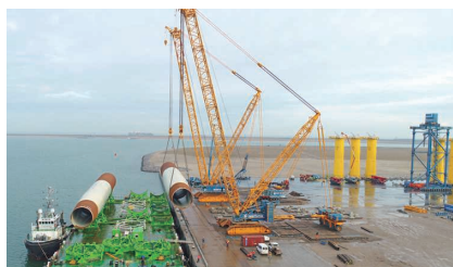
Crawler cranes loading offshore wind turbine components at a port
