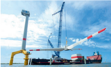
Assembling equipment in the harbor
