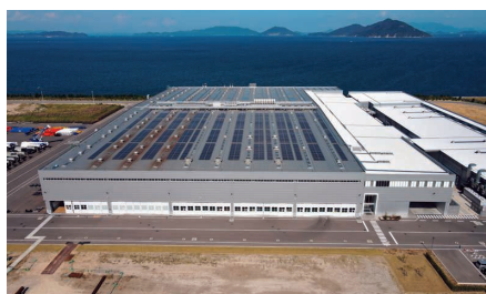
Solar panels installed at Kozai Plant
