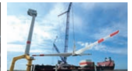
Assembling wind power generation equipment
