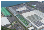
Solar panels installed at Shido Plant
