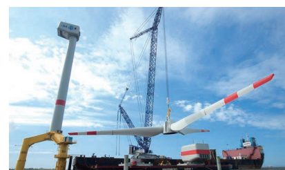
Assembling wind power generation equipment
