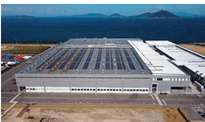
Solar panels installed at Kozai Plant
