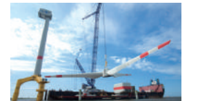
Assembling wind power generation equipment
