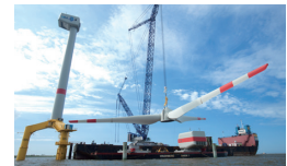
Assembling wind power generation equipment
