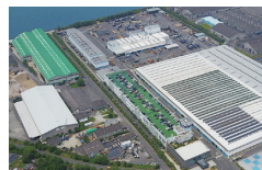
Solar panels installed at the Shido Plant
